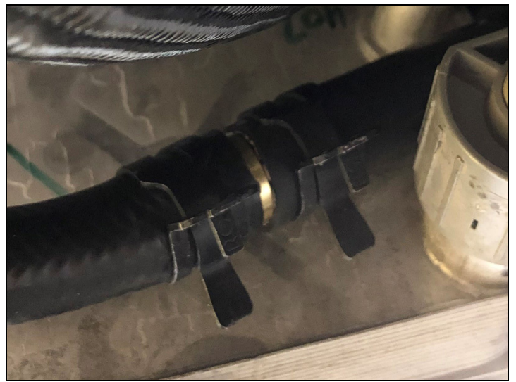
FIGURE 18 – Hose Coupler Installed with Clamps
